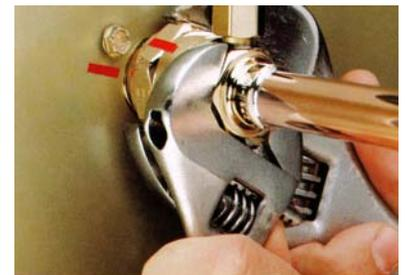
6. After all connections are made, and after the king valve has been opened (do not open at this time) check the couplings for leaks.
