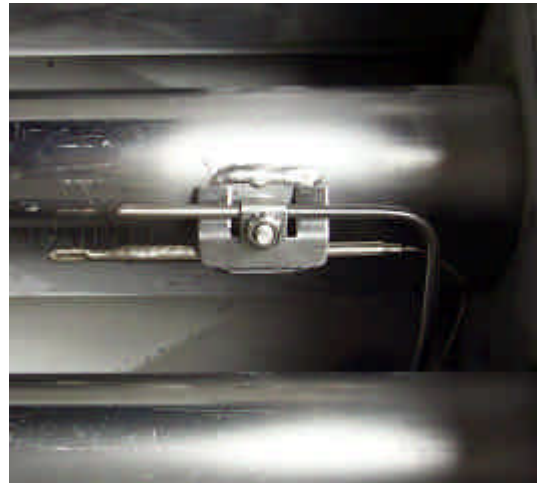
Typical high-limit/sensor probe locations and mounting hardware.
