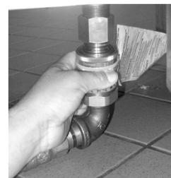
Check both ends of the quick disconnect for grease. Wipe the quick disconnect clean if necessary. Reconnect the gas line coupling.
