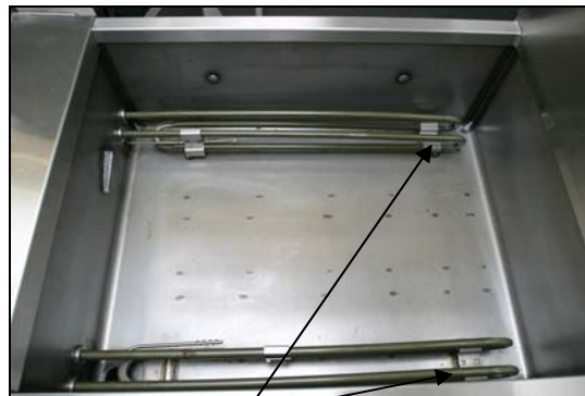
Remove screws here.
