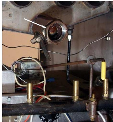
Ball retainer nut (arrow) on drain valve.
