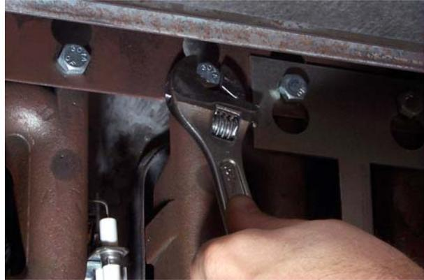
Loosening burner bolts prior to burner removal.
