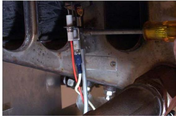
Removing electronic/standing pilot assembly.
