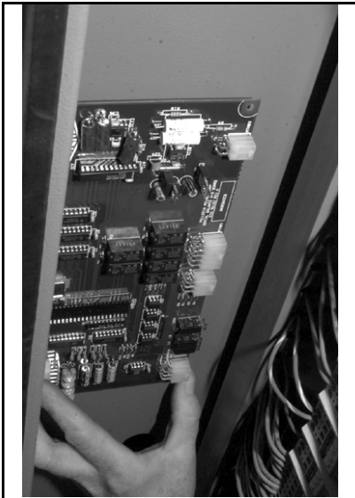
Figure 3: Positioning Balance Board Prior to Installation
