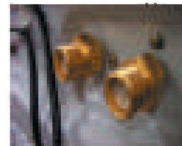
Brass Pressure Regulators installed on back of appliance.
