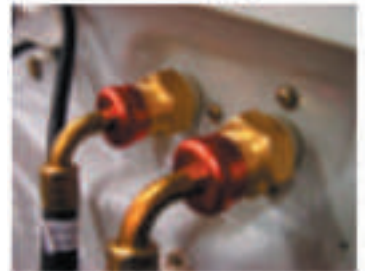
Brass pressure reducers and elbow ends of supply hoses.
