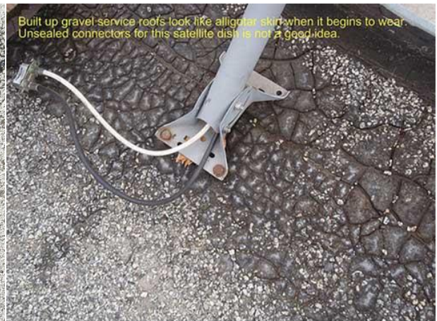
Aged asphalt and incorrect attachment to roof of support leg
