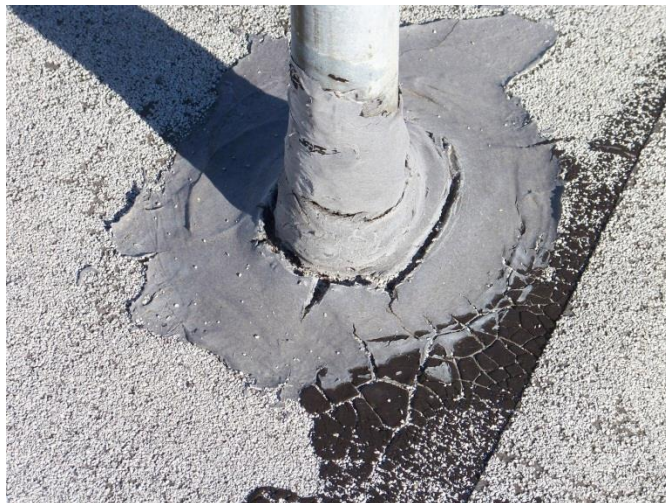
Aged asphalt and incorrect attachment to roof of support leg
