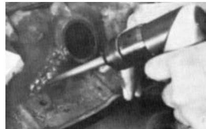
This photo shows a repair with plugs installed and peened ready for resurfacing the casting.
