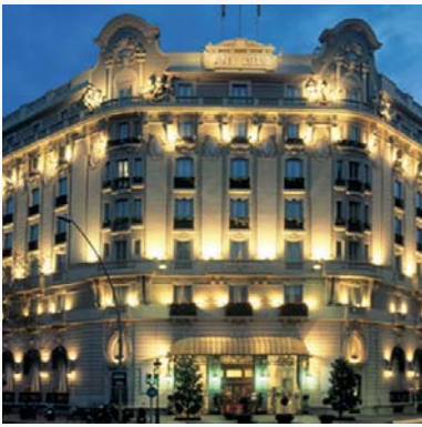
Hotel Palace Barcelona (Spain)
