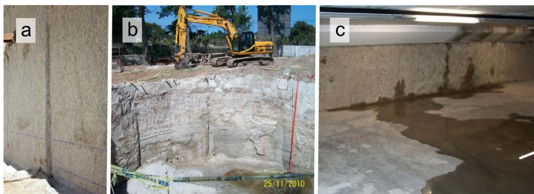
Fig. 1 - Typical defects of diaphragm walls in joints between panels.
