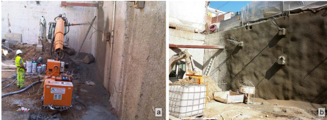
Fig. 8 - Bi-layer walls: (a) Spraying of second layer; (b) finished sprayed surface
