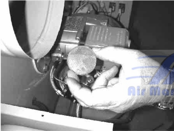
Remove the fuel pump screen
