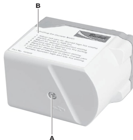
Figure 13A. Damper Motor with Cover
