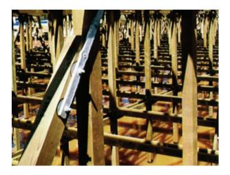
Transverse fan deck and hot water basin girts are  $2'' \times 6''$ —all other transverse girts and all longitudinal girts are  $2'' \times 4''$  except where loading may require  $3'' \times 4''$ . Transverse and longitudinal girts are spaced on 6'-0'' vertical centers. Girt lines are through bolted to the columns.
