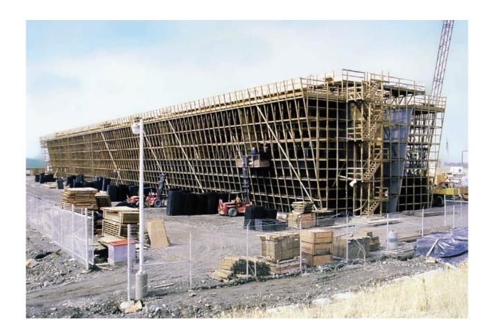
The diagonals brace the structure and carry loads to heavy-duty, hot dip glavanized anchor castings. The anchor castings transmit wind and/or earthquake loads from the structure directly into the foundation.
