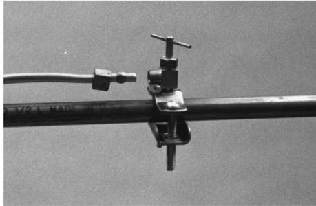
3. Uncoil the copper tubing and connect one end to the saddle valve. Use the compression fittings found in the self-piercing saddle valve parts bag.
