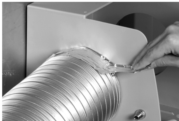
Fig. 15. Sealing connections with tape.
