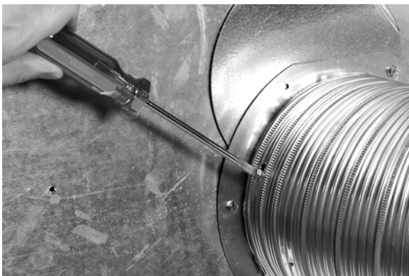
Fig. 13. Connecting Bypass Duct to Bypass Collar.
