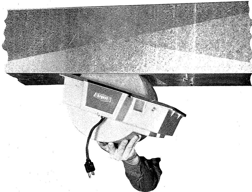
Figure 3—Installing Humidifier
