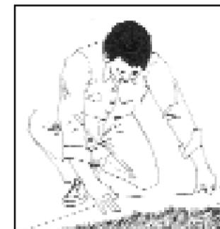
Place cord into trench carefully stretching as you go to remove any twists in cord.
