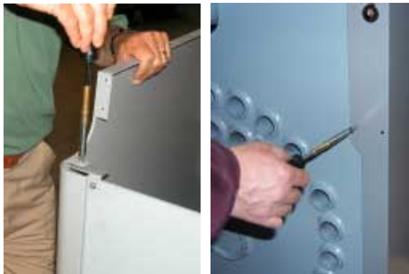
G Secure the sides at the front and rear.
