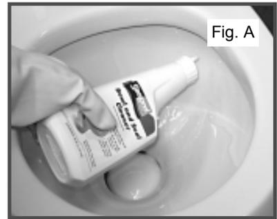
**SEAL CLEANING:** After an extended time, mineral deposits from hard water can build up under the edge of the rubber bowl seal, resulting in a slow leakdown of water from the bowl. To prevent this mineral build-up, periodically clean under the bowl seal with SeaLand Bowl and Seal Cleaner (Fig. B).
