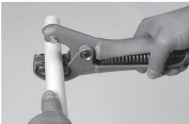
Cut the JRG Sanipex MT pipe to the required length with pipe cutter (art. no. 4836).
