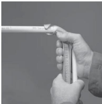
Bending the pipe bend. During bending, the pipe has to be guided as closely along the bending gauge as possible.
