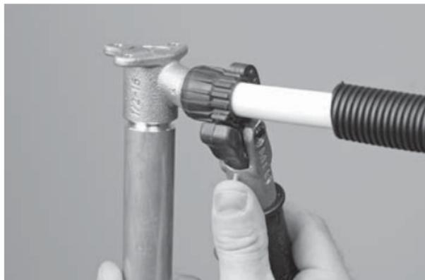
Finally tighten the union nut with the ratchet torque wrench (art. no. 4832). For counter-bracing, use the alignment gauge (art. no. 5777) or the counterung spanner (art. no. 4834).
