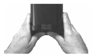
To mount the cover proceed to insert the bottom part a few cm. under the bottom plate so that it fixes into the guides of the aluminium section which makes up the rack. Press the cover from the bottom towards the top so that by sliding it along the guides it snaps into the top plate, then screw tight to fasten.
