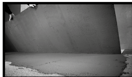
Fig.68 - 2 - Rest the slab on its long side and guide it towards the floor.
