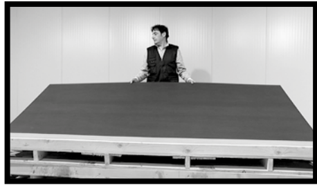
Fig.1 - All types of 300x100 cm slabs of KERLITE can be lifted by one person only. Lift the slab with open hands. Slowly raise the longer side so as to eliminate the suction effect, due to contact with the underlying slab, and ensure a good grip.
