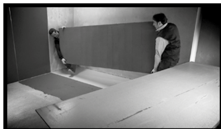
Fig.67 - 1 - To handle slabs, raise them to their upright position, whilst grasping them from the top edge. Move the slabs keeping them straight and with the aid of another person.
