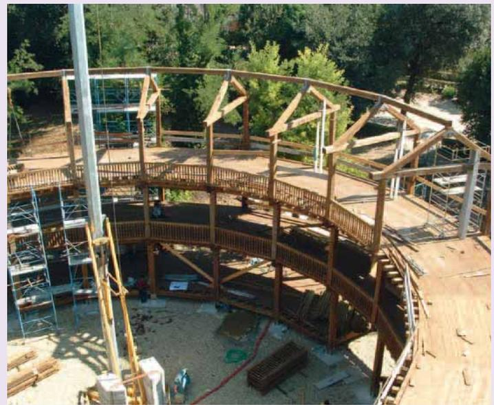
so that the theatre can be taken apart and put back together on another site, or its components can be recycled and reused. The Silvano Toti Globe has no solar or photovoltaic panels, but should in any case be considered one of the newly built projects standing out the most for its focus on the issues of environmentally compatible and sustainable construction. The proof of this is its complete removability, potential
