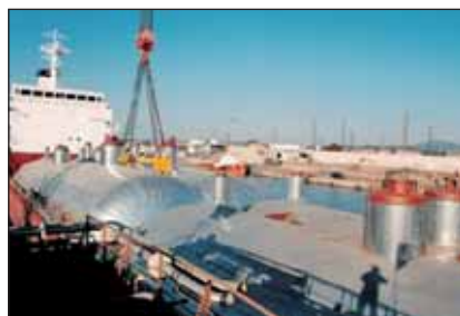
Figure 8 - Bi-lobe type C tank during lifting on board.
