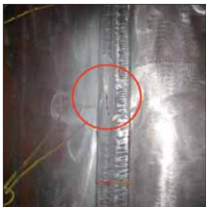
Figure 18 - View of dye penetrant test on defect shown in Figure 17 after excavation.
