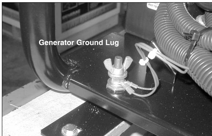
Figure 13 - Grounding the Generator
