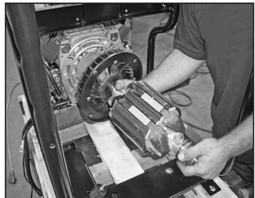
Figure 7-9. – Remove Rotor
