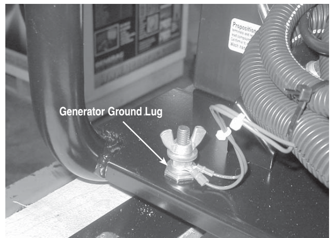
Figure 13 - Grounding the Generator
