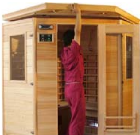
FIG-16 Assembling internal top board
