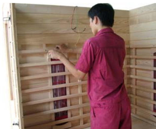
FIG-13.1 Fixing backrest with screws
