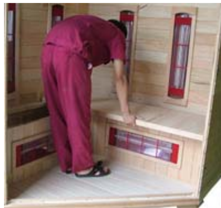
FIG-12 Assembling sitting board
