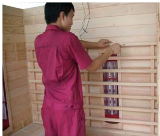
FIG-13 Fix the backrest with screws
