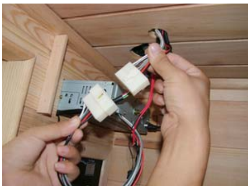
FIG-20 Link the CD connectors
