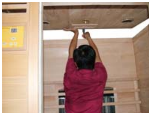
FIG-17 Leading the wires of heaters onto the board through the corresponding hole
