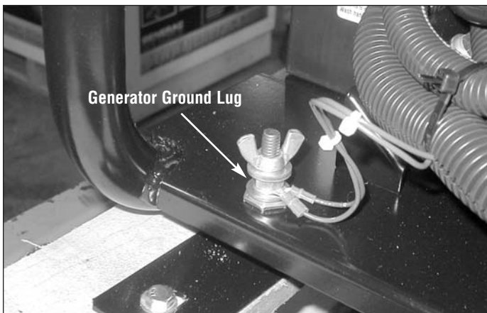
Figure 13 - Grounding the Generator
