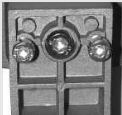
Fig. 47: Cradle adjustment screws.
