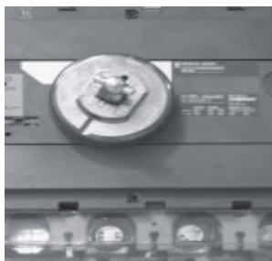
Interruptor LIGADO/DESLIGADO principal
