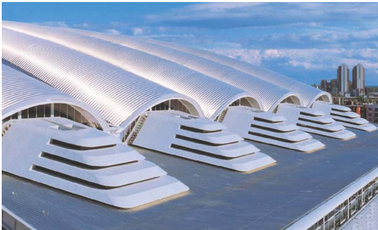
Feira de Frankfurt, Hall 3, Alemanha Arquitecto: Nicholas Grimshaw & Partners
