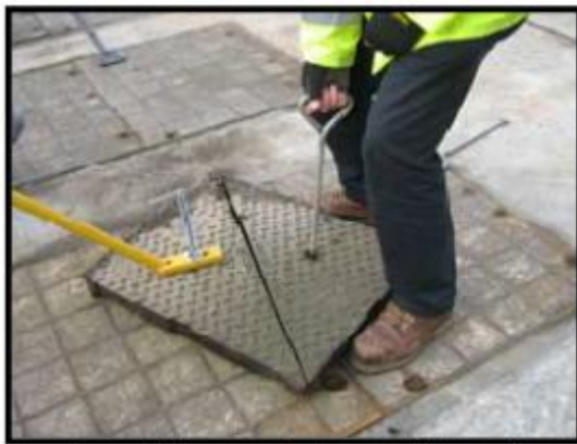
(use of manhole key not allowing good lifting posture)
