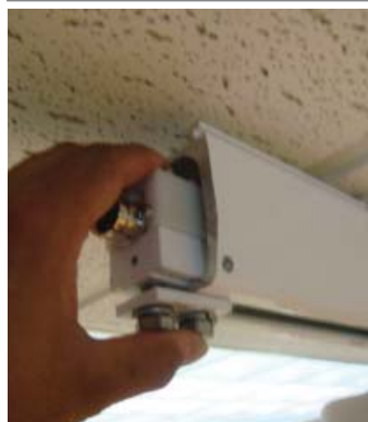
1.7 Remove end stop block and plate
