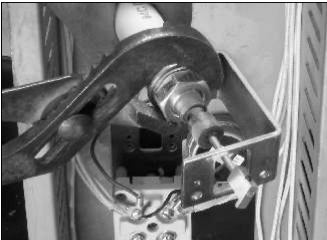
Tighten the nut on the Dawson tube assembly.
