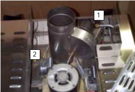
Photo 10 Flue Assembly
