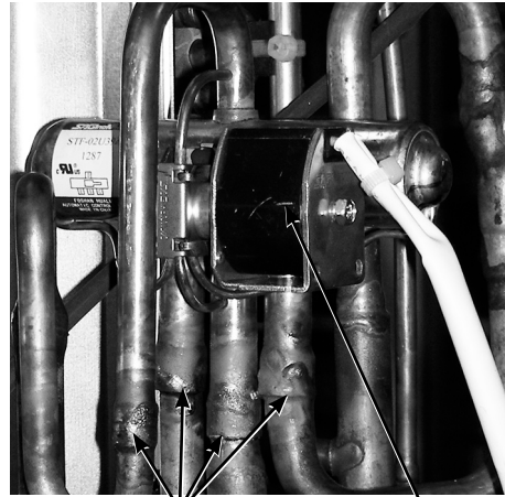
Brazed parts of 4-way valve R.V. coil
