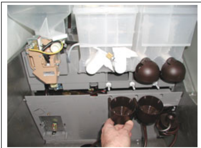
Removal of wall for access to electric mixers
