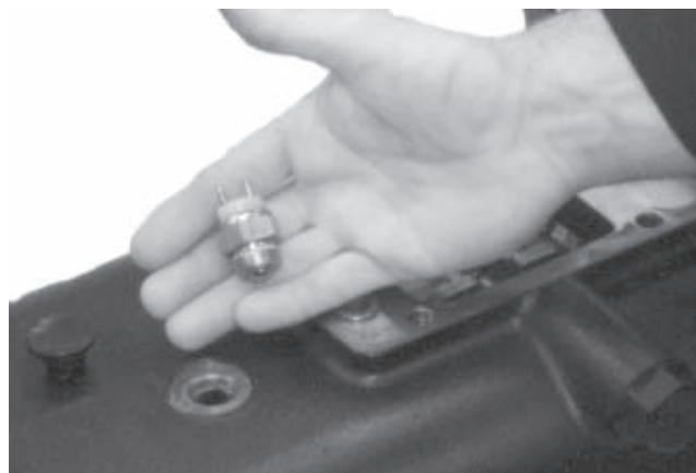
21. Install the backup light switch if it was removed earlier. Torque it to 25 - 41 ft. lbs.
