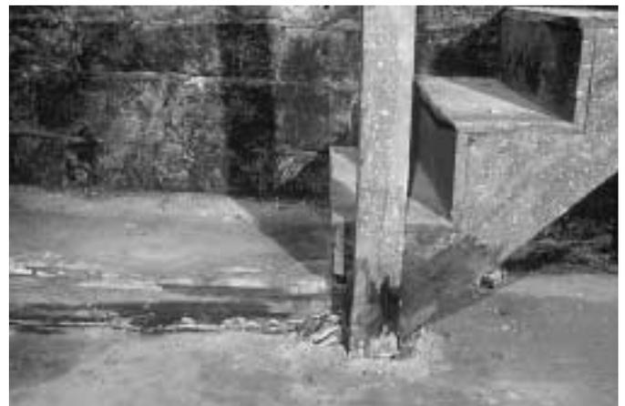
**Figure 3.14.** To prevent termite infestations, do not allow wood form boards to be embedded in concrete as shown in this basement.
