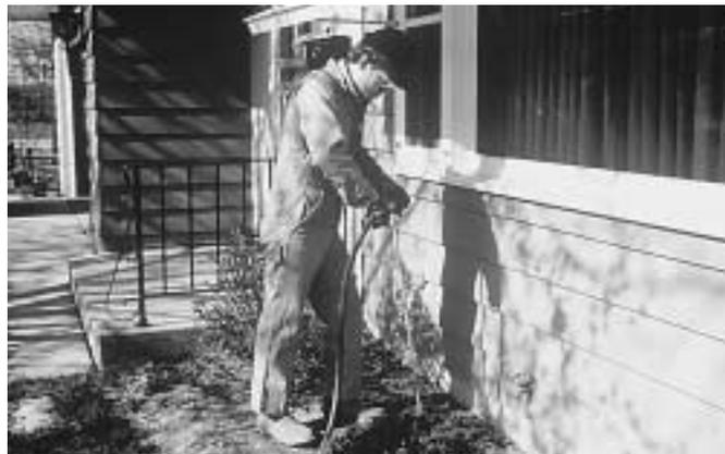
Figure 3.3. Pest management professional applying termiticide to the soil by long rodding the exterior of a house.
