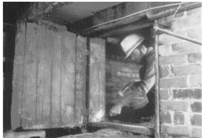
**Figure 3.9.** Inspection of crawl space for termite infestations (he should also be wearing gloves).
