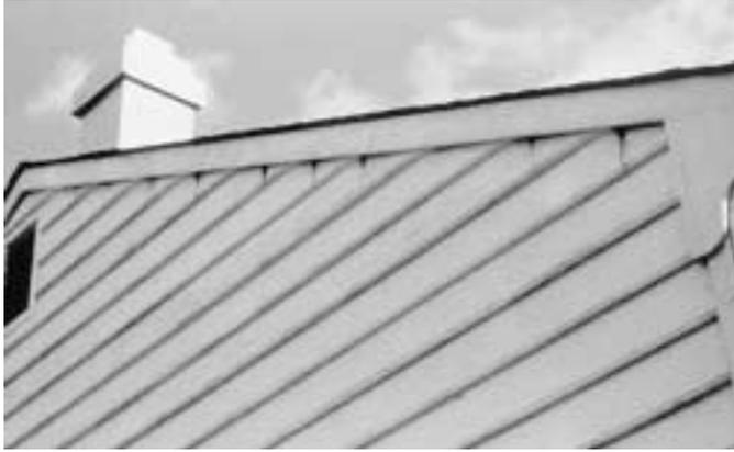
**Figure 6.20. Carpenter bee damage.**
