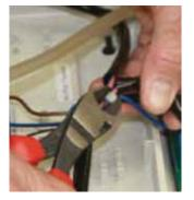
**5** Using Wire Clippers (or a sharp knife) carefully cut and remove the cable tie securing the power leads between the two halves of the unit.
