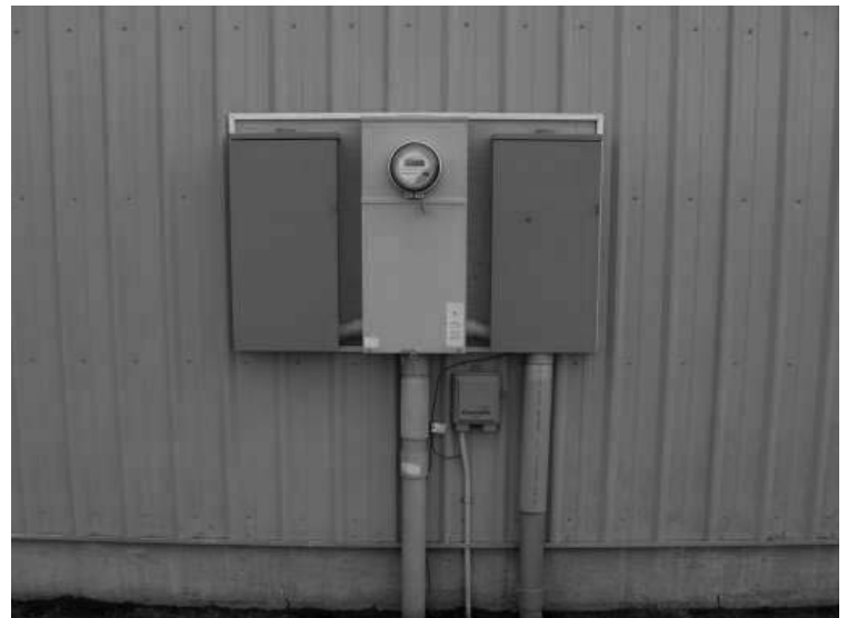
FIGURE 1-15b 320 amp Surface mounted meter socket
