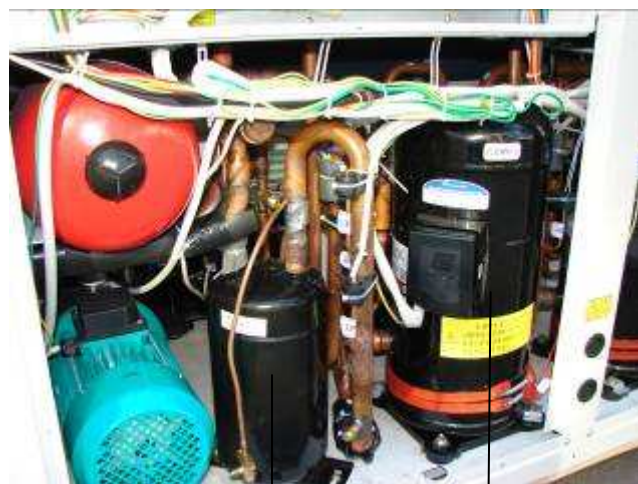
Gas-liquid separator
