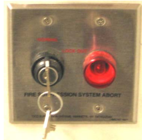
Figure 21: Maintenance Switch
