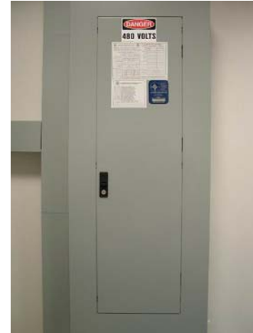
Figure 26: 480V AC Electrical Panel
