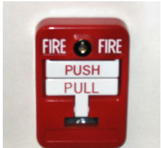
Figure 18: Fire Alarm Pull Station
