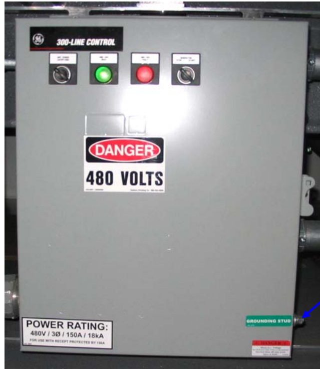
Figure 28: Ground Connection
