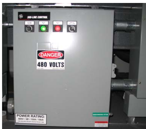
Figure 24: 480 V AC Electrical Control Panel
