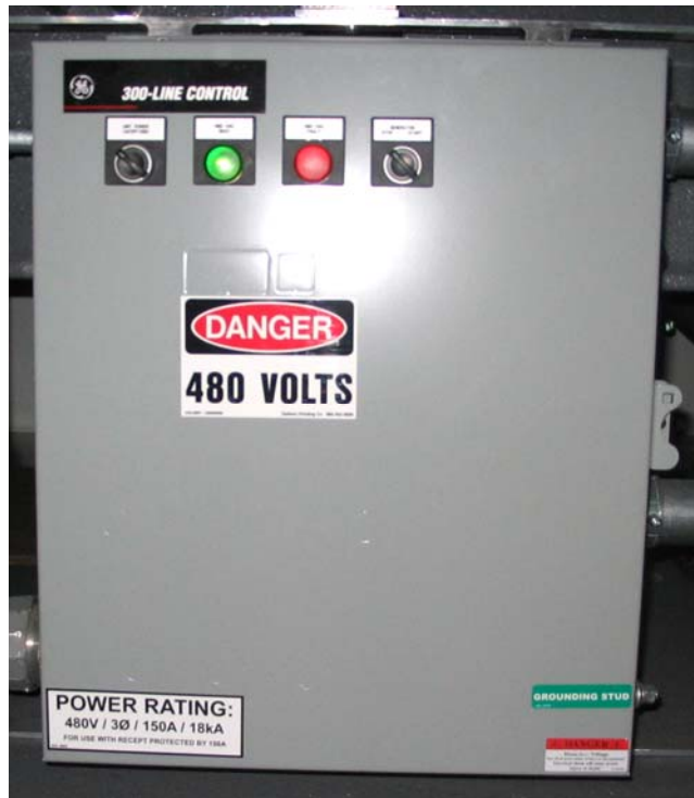
Figure 44: 480V AC Fault Indicator Light
