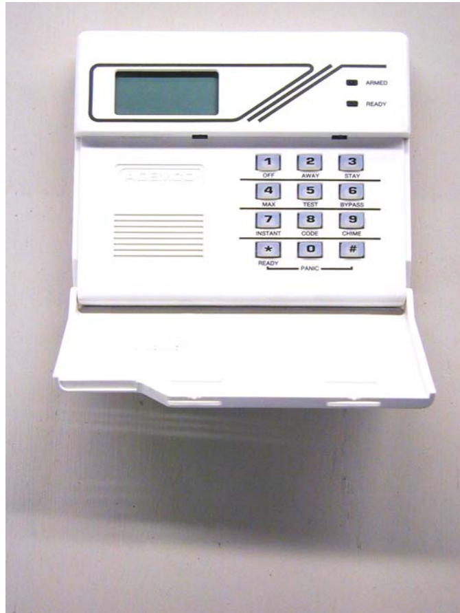
Figure 37: Intrusion Alarm Keypad
