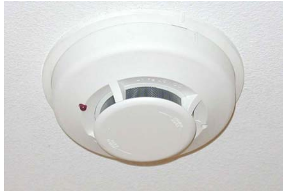
Figure 16: Smoke Detector
