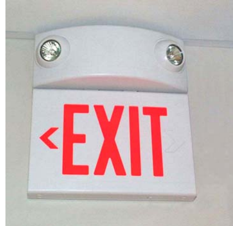
Figure 40: Emergency Dual Beam Lighting
