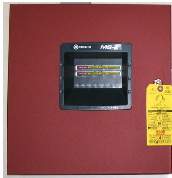
Figure 17: Fire Alarm Control Panel
