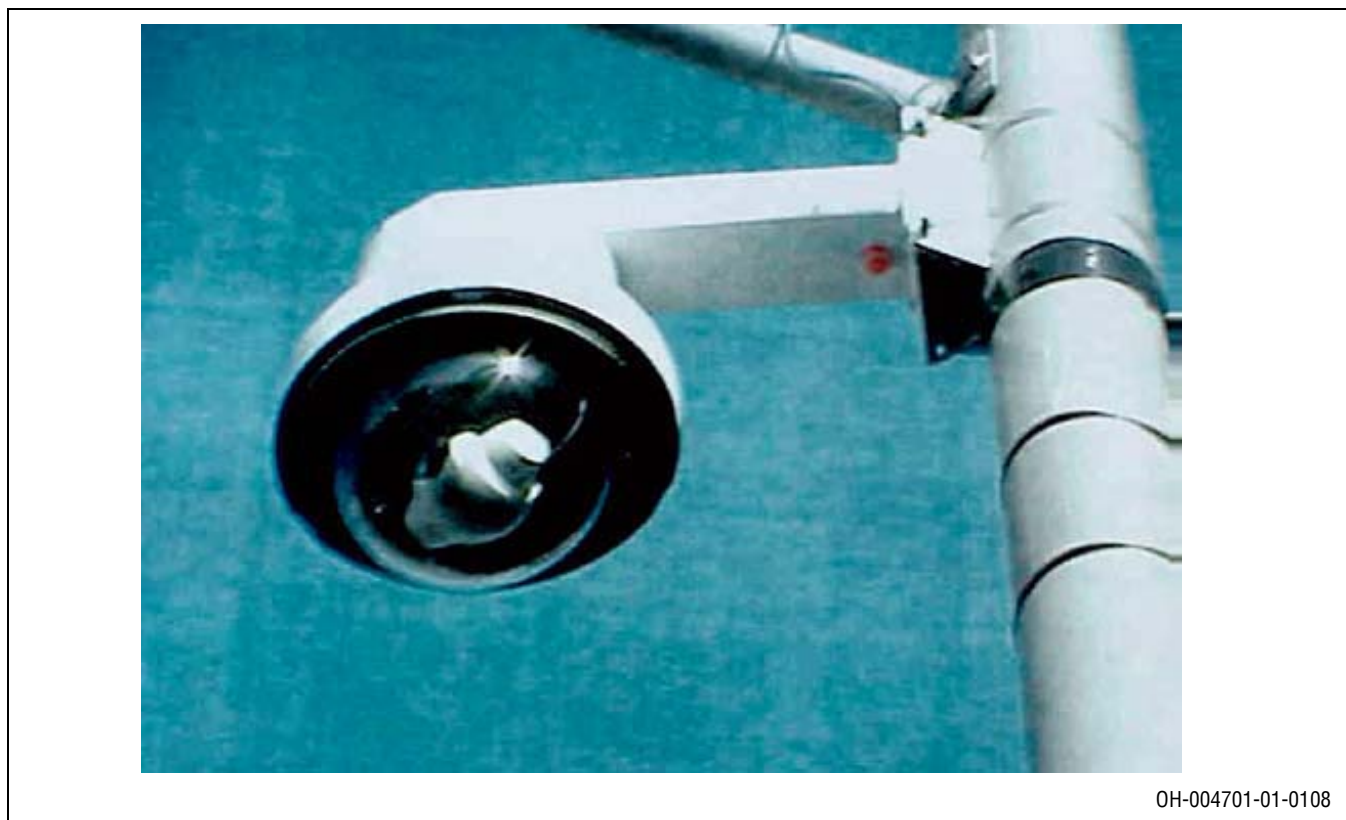
Figure 6.4: Camera Attachment to Metal Pole
