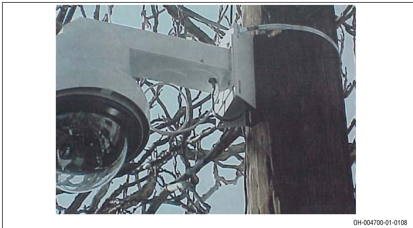
Figure 6.4: Camera Attachment to Metal Pole
