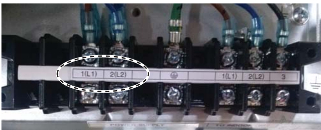
< Input Power Source Check Point >
