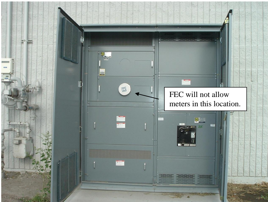
Photo 6: Switchboard Cabinet
