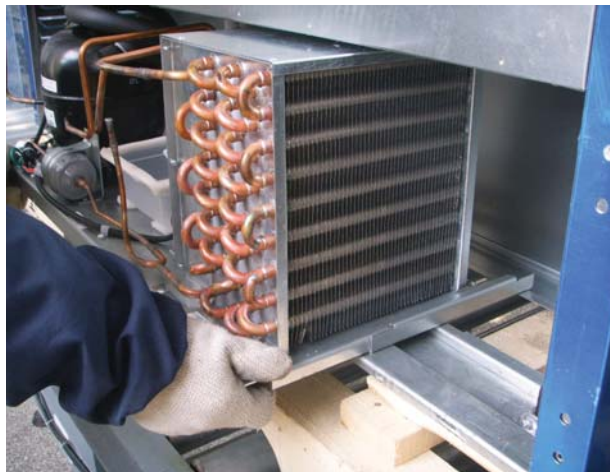
Pull out the condensing unit
