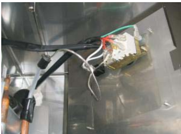
E. Remove the thermostat & sensor
